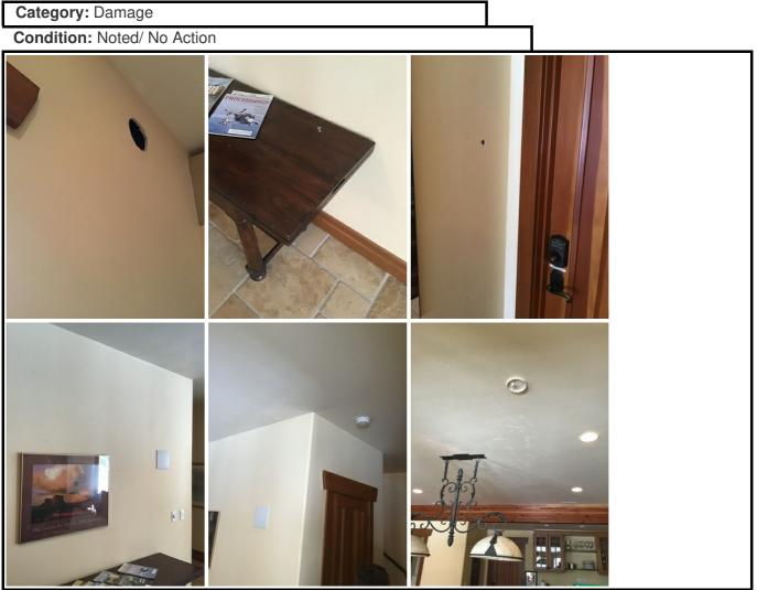
**Comments:** - Remove extra smoke alarm mount, patch and paint. - Minor patch and paintwork left of hallway exit. - Large hole and 2 small holes in the wall left of the door with a keypad. - Blue paint on the long brown table as you enter the dining area from the hall. - A big hole in the drywall in storage behind the kitchen area.
