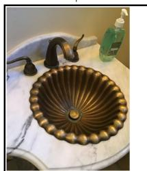
**Comments:** - the sink drain stopper does not seal completely when closed water is still draining.
