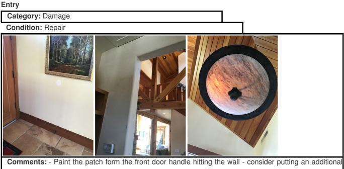
doorstop where the handle could hit - Check hanging fixture for a potential 1 or 2 bulbs out - 2 chips on the archway to bathroom. Cleaning will remove most marks but some need a paint touch up
